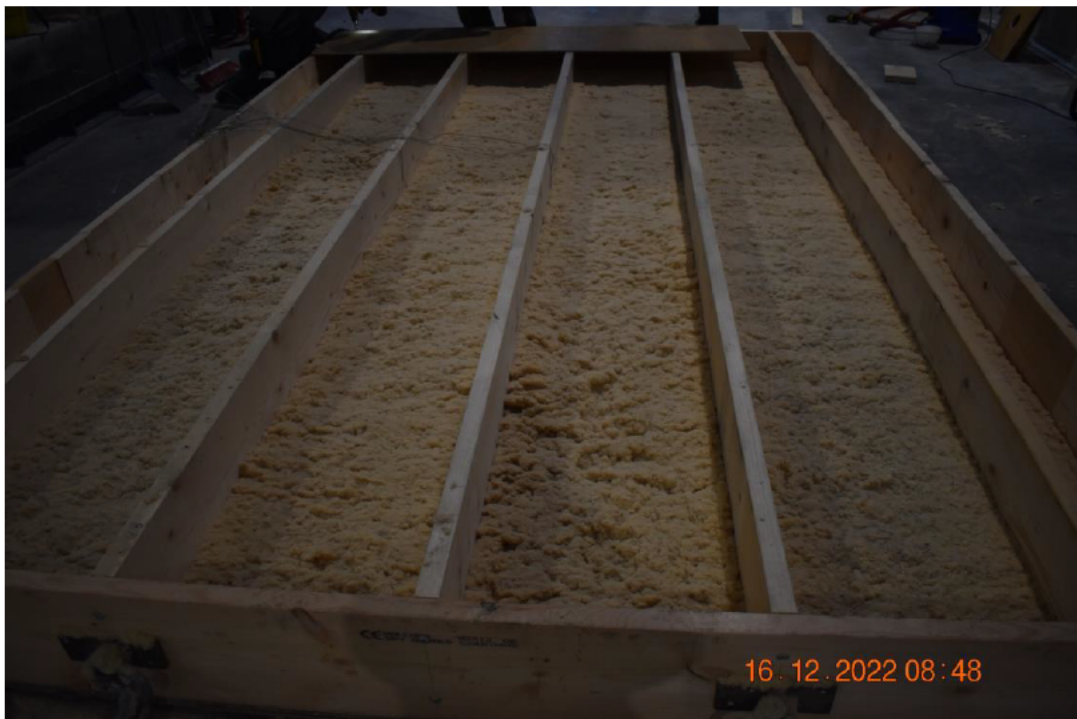
Photo No. 8 Insulation of construction
