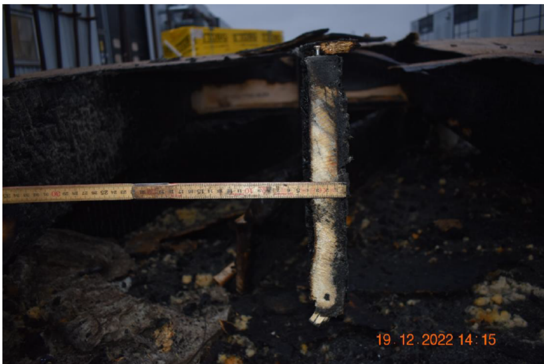
Photo No. 18 Loadbearing beams after the test
