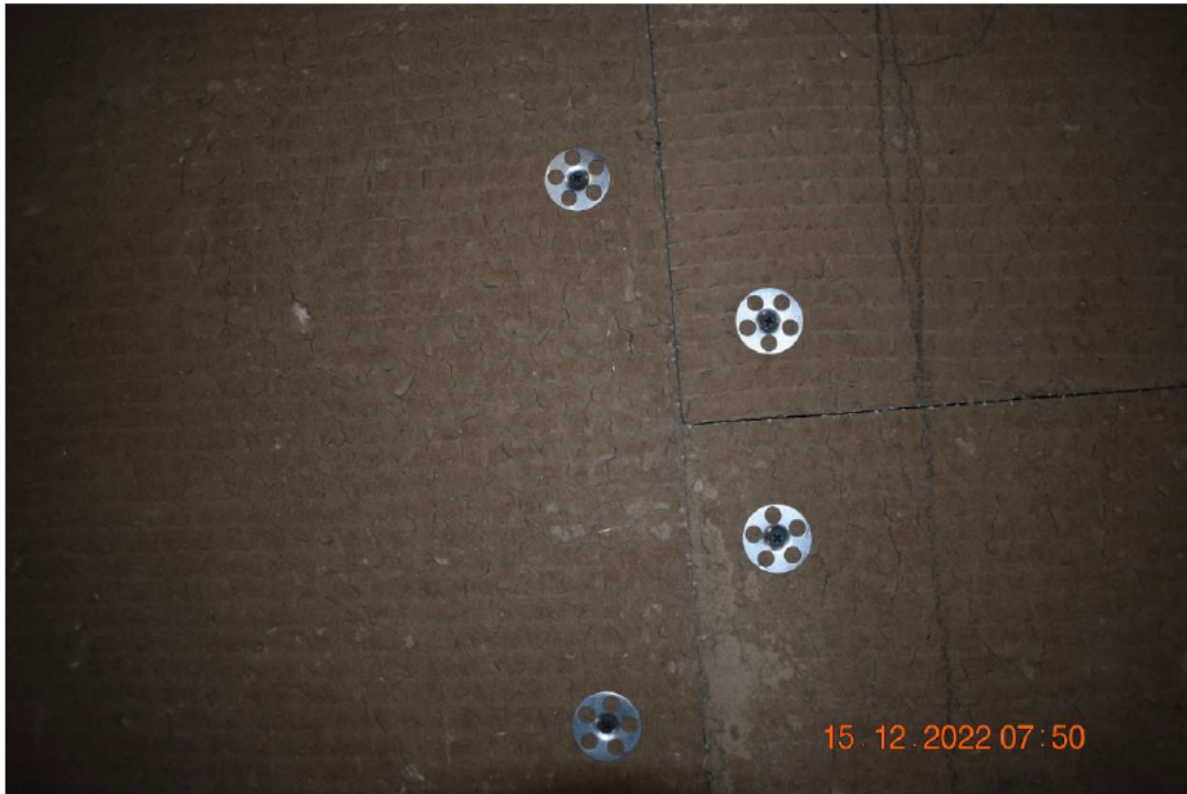
Photo No. 5 Washers for 2 nd layer of clay boards
