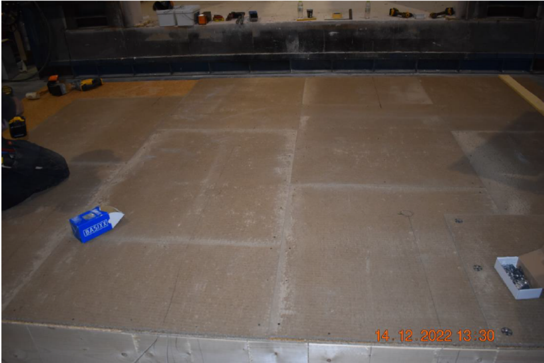
Photo No. 3 1 st layer of clay boards
