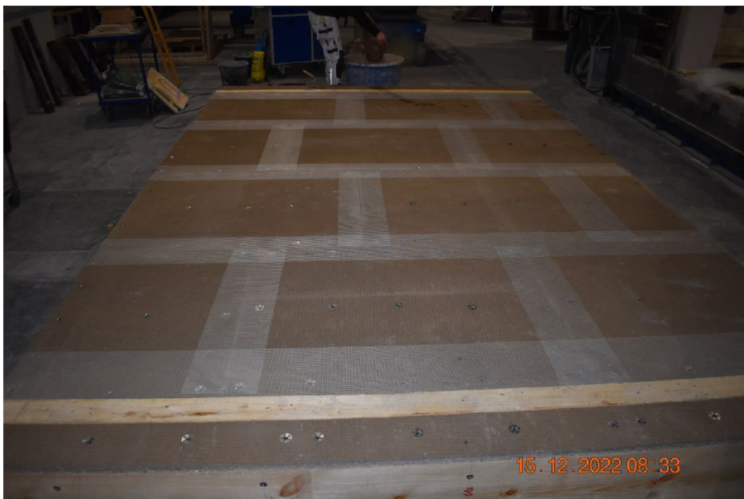
Photo No. 6 Reinforcement mesh before application of clay plaster
