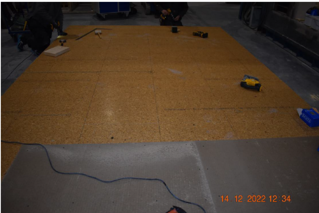
Photo No. 2 Bottom layer of chipboard
