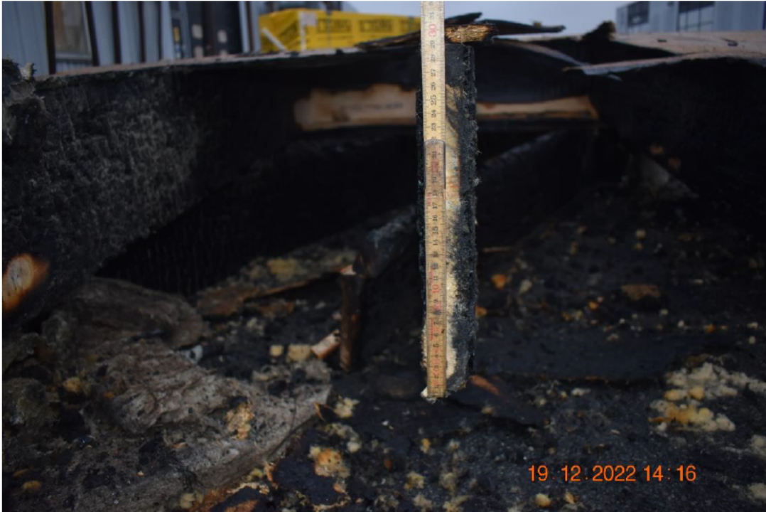
Photo No. 19 Loadbearing beams after the test
