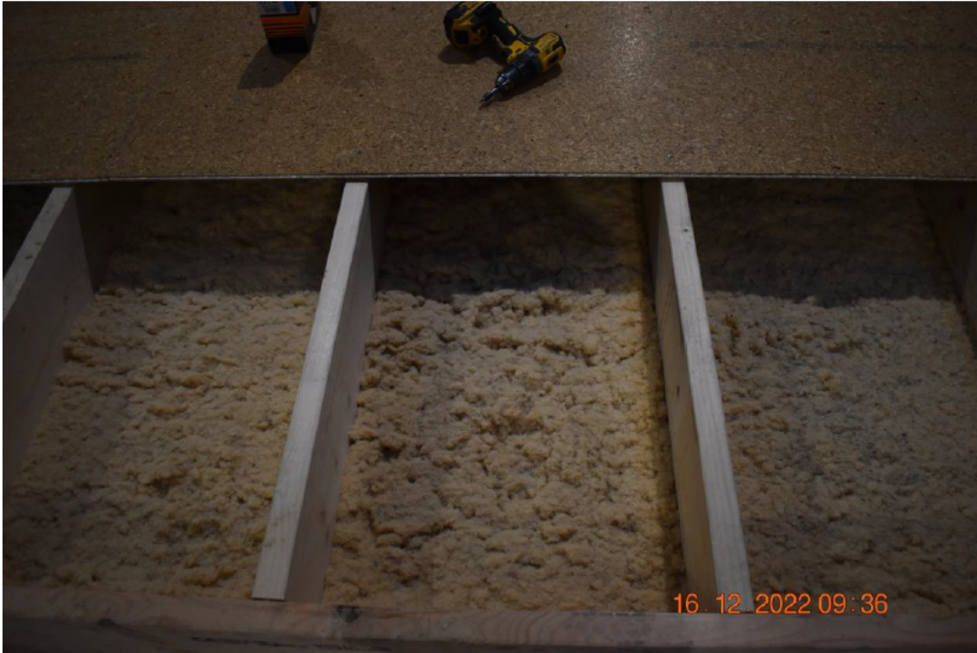
Photo No. 9 Chipboard installation on unexposed side
