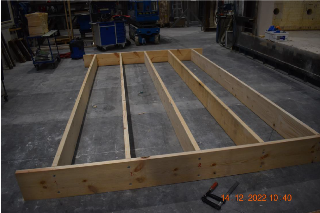
Photo No. 1 Loadbearing beams during mounting
