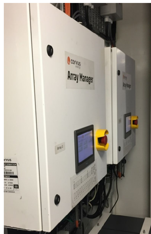
Photo 4. The Corvus Array Manager monitors the batteries and temperatures. The only way for the crew to access the batteries is via the touch screen on the front of the box.
