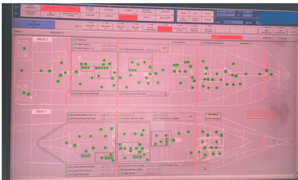
Photo 9. A digital overview of all alarms, including fire alarms, on one of the decks. In total there are 8000 various alarms to consider in the "Hybrid" system and 5-6000 in the "Electric" system.
